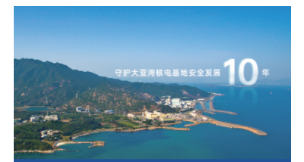
World's First Nuclear-grade Backup Power Plant Shenzhen 2.5MW/3.5MWh
