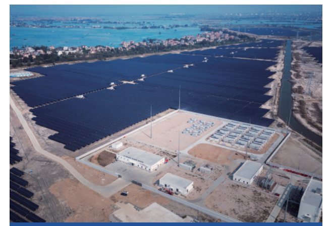
High Temp./Humidity/Salt Fog First Salt + PV Complementary Project Hainan 25MW/50MWh
